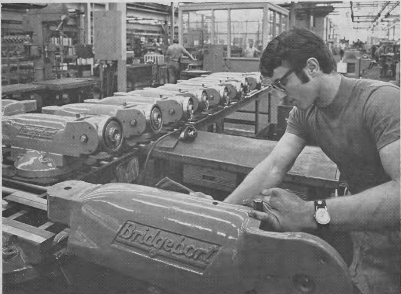
Ram is assembled to turret after wiping down dovetails (above) in line that feeds into three main assembly lines (right) where completed machines are built up. Machines move on wheeled pallets
